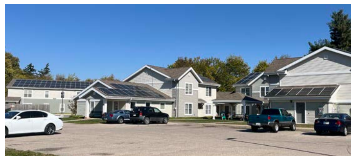
ABOVE: Installed solar panels on our apartments at Westplains in Goshen.
