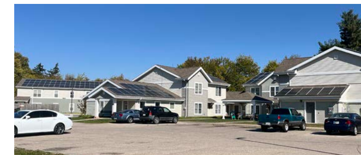
ABOVE: Installed solar panels on our apartments at Westplains in Goshen.
